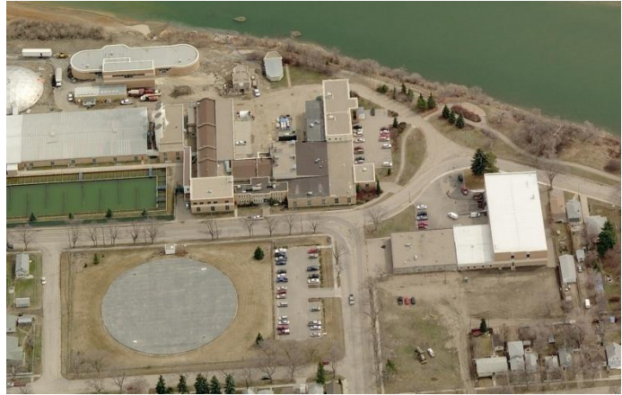
Aerial view of Water Treatment Plant and Meter Shop – Avenue H South
