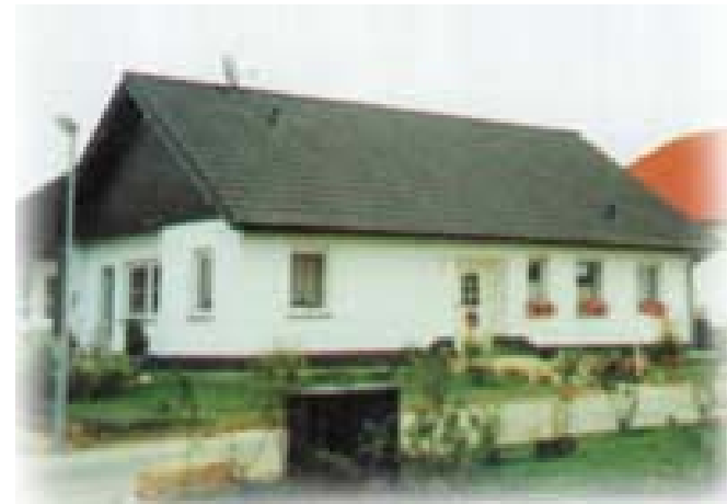
Figure 15 Example of Unacceptable Large Roof Areas
