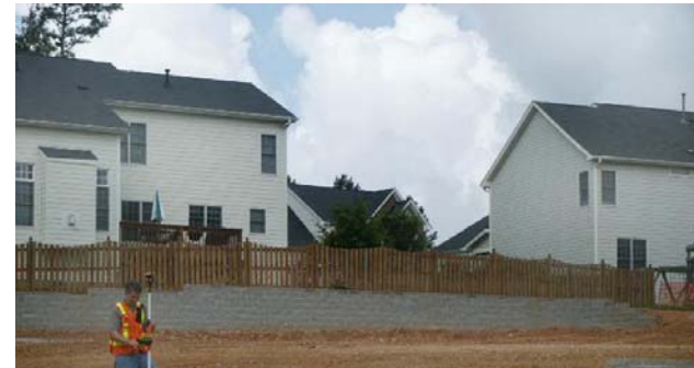
Figure 6 Poor Example of Wall Cladding Variety
