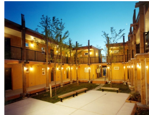
Figure 20 Example Site & Building Lighting
