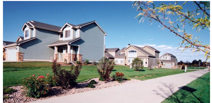
Figure 12 Example of blank walls without Fenestration
