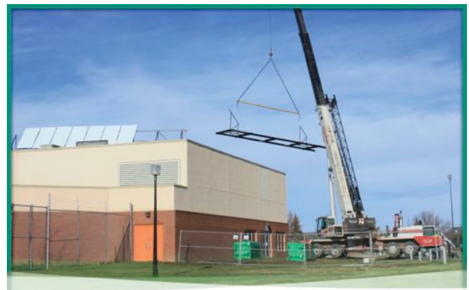
Installation of solar panels at the Lawson Civic Centre
