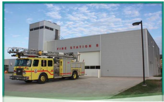
The newly opened Fire Station #8
